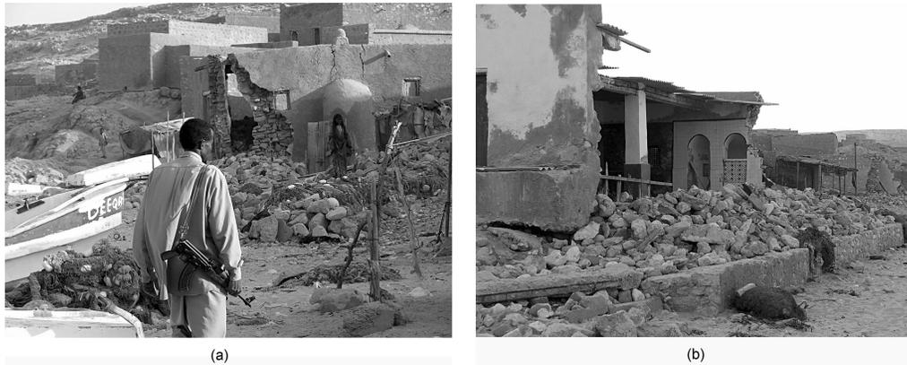
**Figure 6.** Bandarbeyla: (a) a destroyed rock house corner and an armed bodyguard leading the way; (b) blowout failure of walls parallel to the shoreline.
