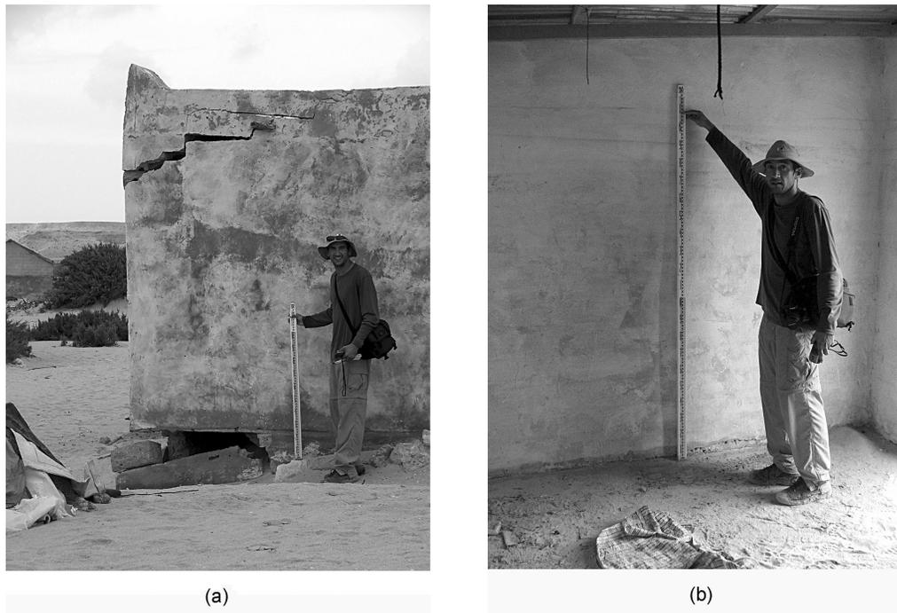
**Figure 11.** Xaafuun: (a) scour damaged a house corner; (b) a flow depth recording based on a watermark on a house wall.
